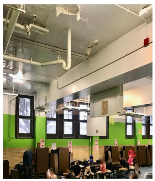
Photo 3 – Occupied "Cafetorium" (gym and lunchroom) — Kids sitting and eating underneath severely damaged lead painted ceiling
