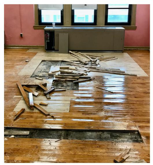
**Photo 9 – ES Classroom —** Repeat flooding from malfunctioning classroom unit ventilator resulting in extensive damage and mold growth to newly installed flooring — the original flooring was replaced for the same reason just a few weeks earlier. An example of what happens if the "root causes" are not addressed and also issues related to inadequate governance, oversight, and management
