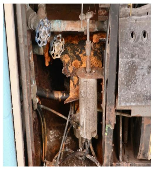
**Photo 16 – ES – Classroom Unit Ventilator -** Typical *inside* condition of the CUVs [dirty, rusted, leaking, & deteriorated with mold & bacterial slime]
