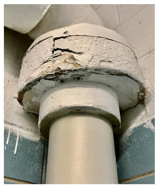
**Photo 19 – Bathroom (close-up of above) —** Showing damage to asbestos insulation
