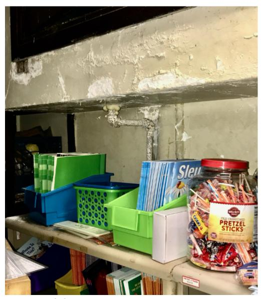
**Photo 4 – ES Closet —** Food and books stored where lead paint is flaking with dust and debris on materials
