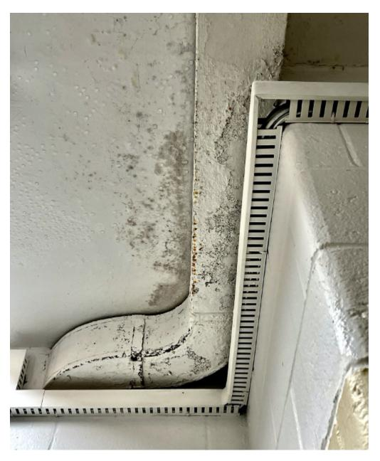
Photo 8 - **ES Bathroom** – Mold growing on ceiling and ductwork
