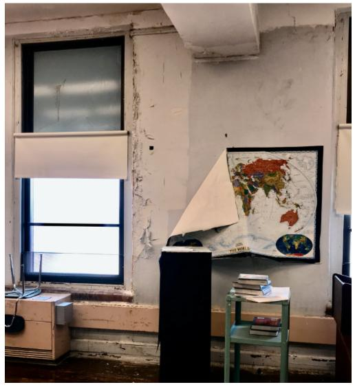
**Photo 1— ES Classroom —** Antiquated classroom unit ventilator, damaged/flaking lead paint, and obvious signs - and damage associated with - moisture and water intrusion.
