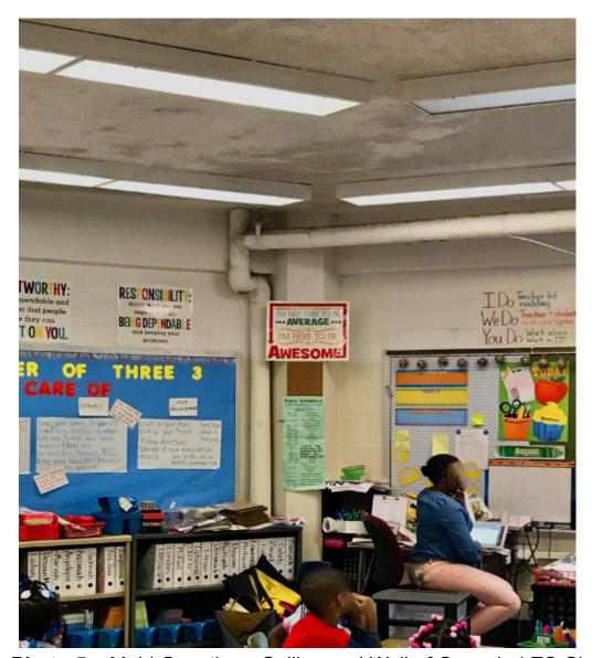
**Photo 5 –** Mold Growth on Ceiling and Wall of Occupied ES Classroom (close up of above) — According to Classroom Teacher This Condition Had Been Present for Several Months — Associated with HVAC System Problems
