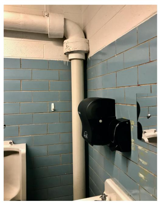
**Photo 18 – Bathroom —** Accessible, damaged asbestos insulation between urinal and sink — this condition is present in multiple locations
